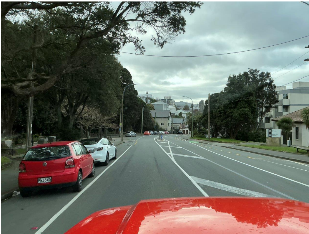
Figure 14: Ghost Marking on Pavement - Part 3
