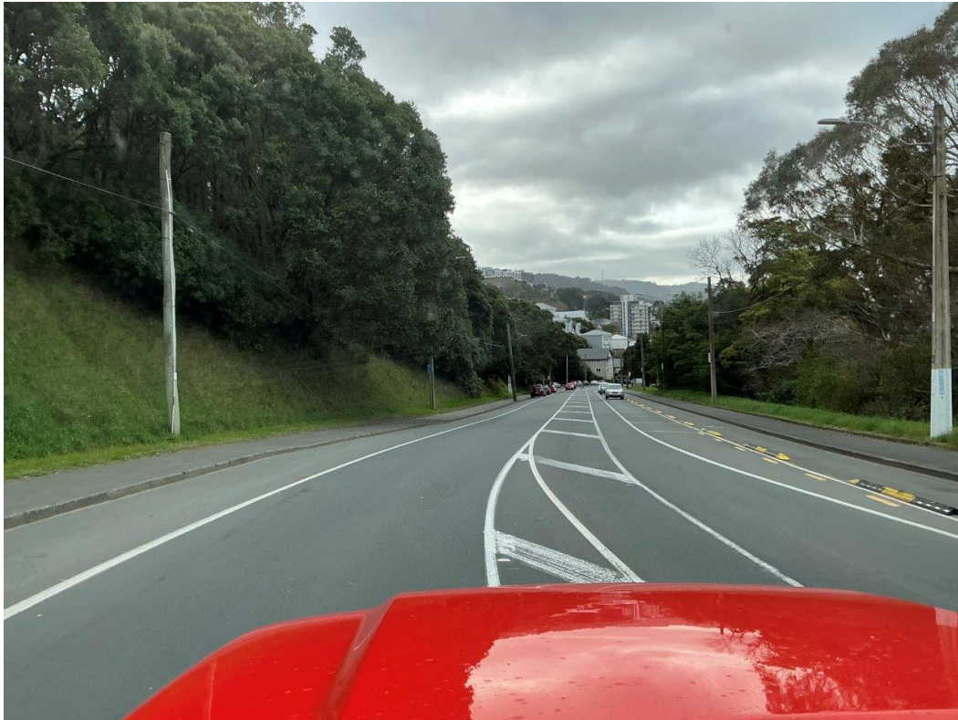
Figure 13: Ghost Marking on Pavement - Part 2
