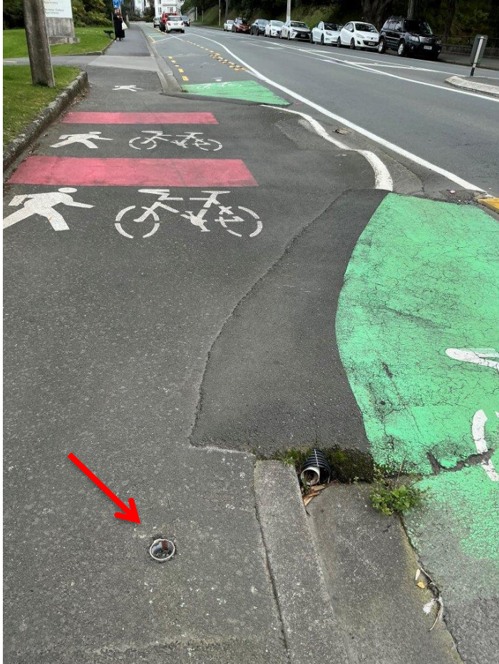
Figure 11: Exposed Sign Post Hole
