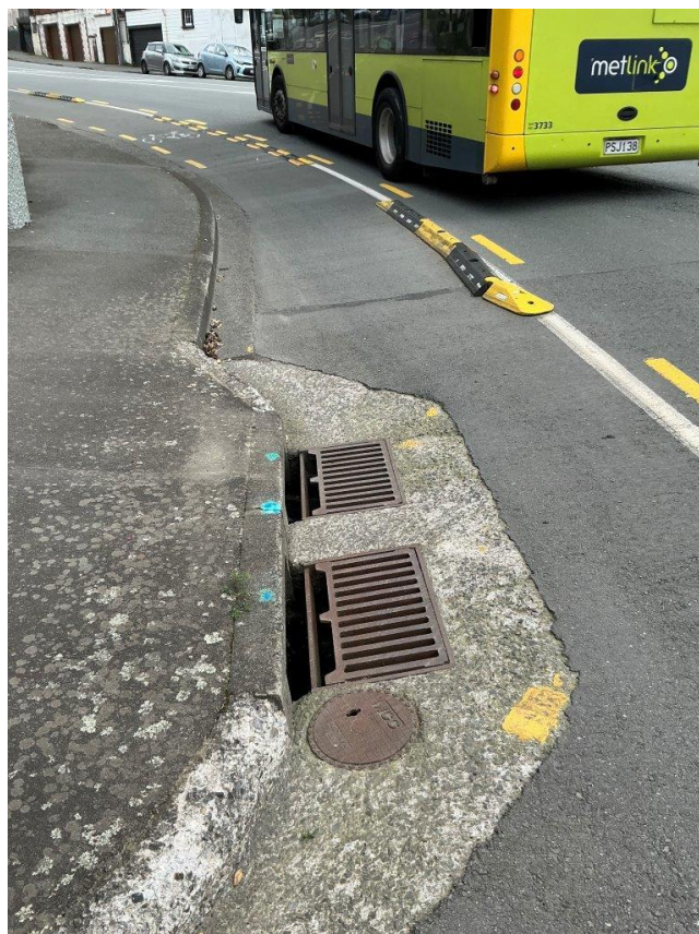
Figure 10: Stormwater Sump on Cycle Way – On-site
