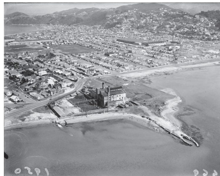
1950 Evans Bay power station shut down in 1968. Original remnants of point remains
