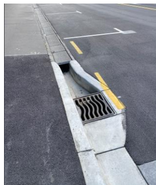
Figure 3-3: Gap left between steel plate for storm water
