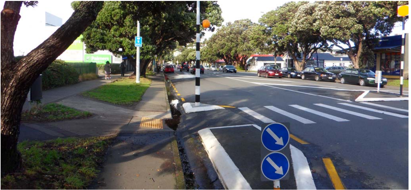
Figure 3.20: Miramar Avenue midblock zebra crossing and kerb build outs between Stone Street and Tauhinu / Portsmouth (facing east)
