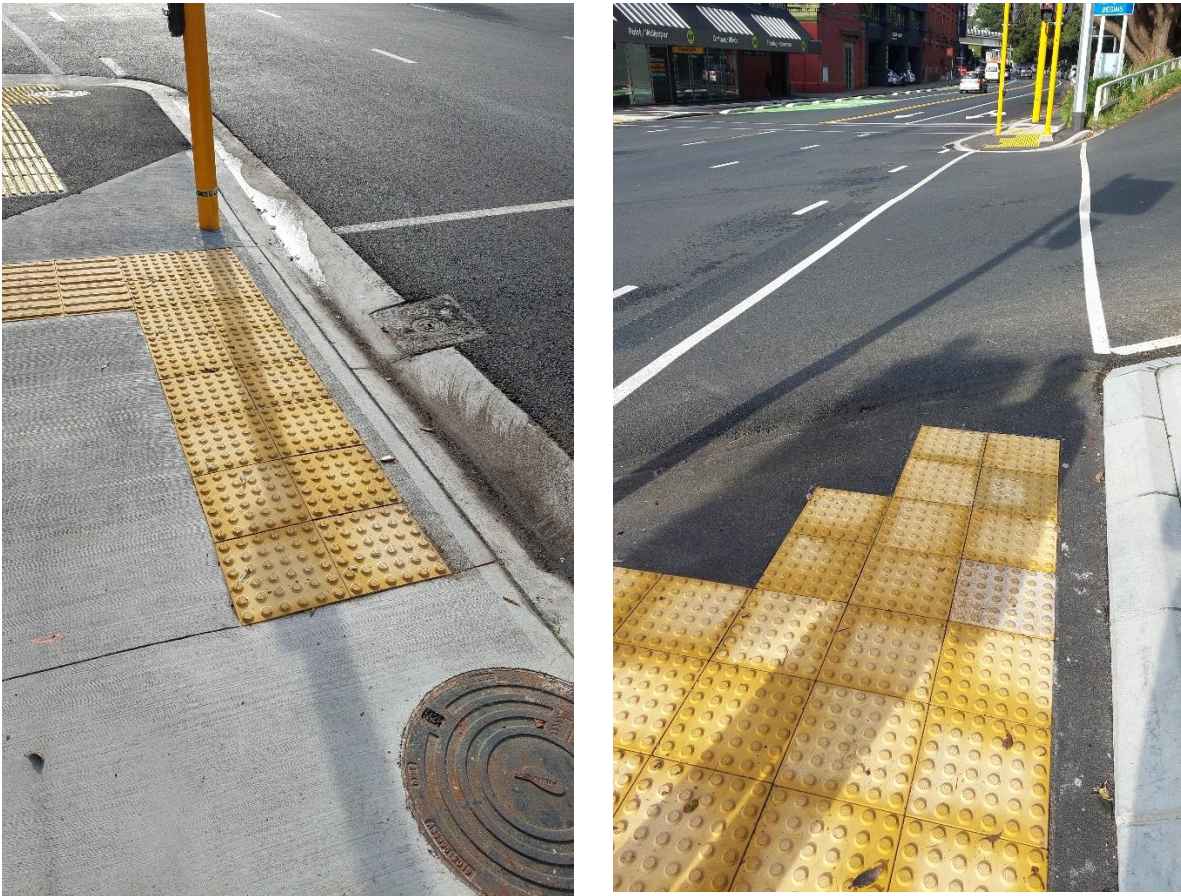
Figure 8. Tactile pavers at Tinakori Road
