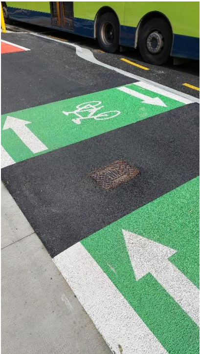
Figure 9. Service cover at Guthrie Bowron that is not flush
