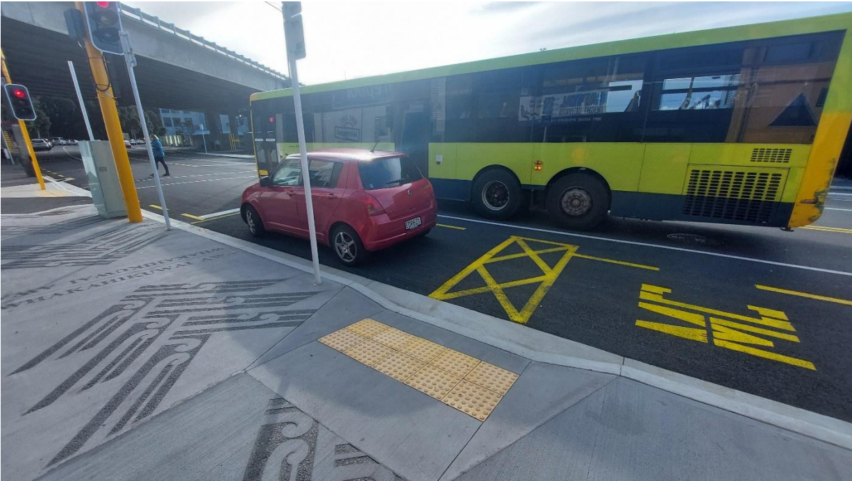
Figure 12. Tactile pavers at mobility carpark.
