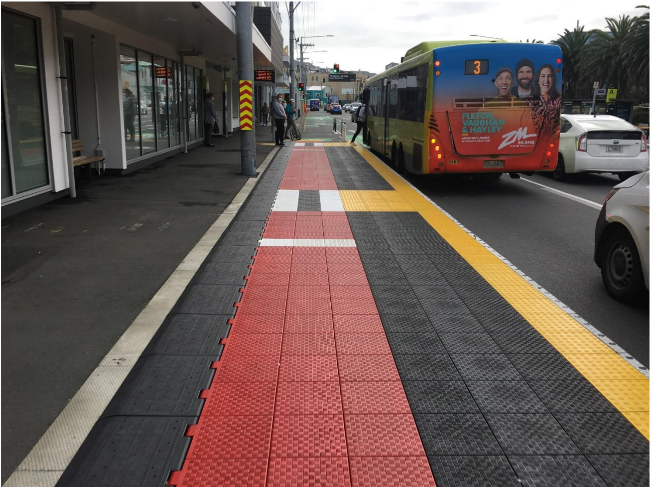
Figure 4: Northbound bus stop platform
