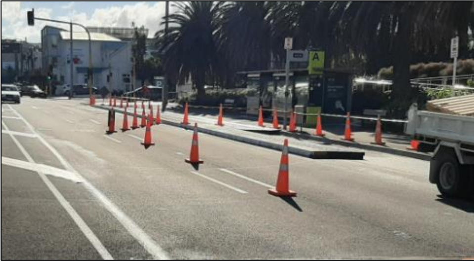
Figure 2 Zicla bus stop being installed outside the hospital for the Newtown to City Transitional Cycleway
