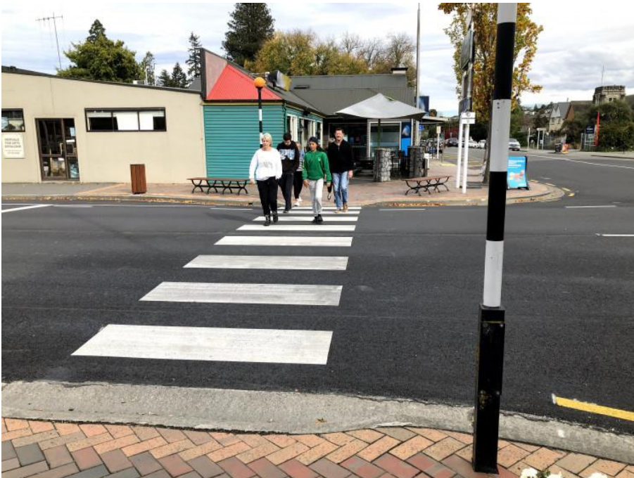
Figure 3.3: Example of a pedestrian zebra crossing (Source: Waka Kotahi, Pedestrian Network Guidance)
