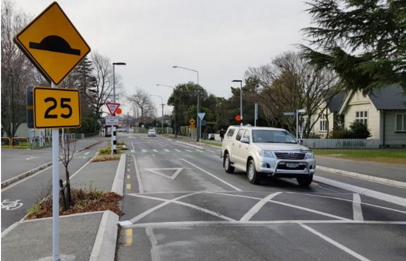
Figure 3.2: Example of vertical deflection (Source: Waka Kotahi, Cycling Network Guidance)
