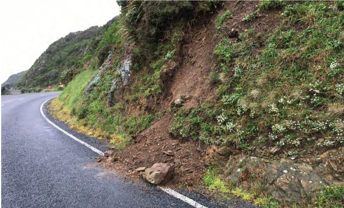
Figure 5: Shallow slide of loose surficial soils and rock observed on 19 June 2020. Approximately 1 m 3 debris inundating road shoulder
