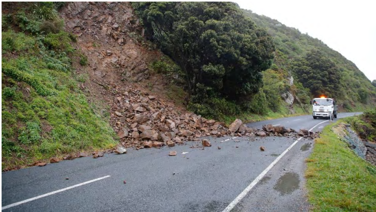
Figure 6: Rockmass slide at CH 1100 m on 19 June 2020 blocking the road (photograph sourced from stuff.co.nz )
