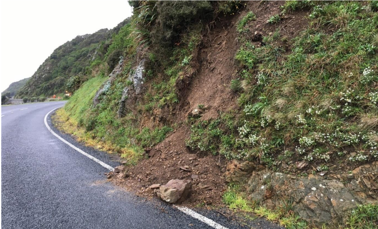
Figure 5: Shallow slide of loose surficial soils and rock observed on 19 June 2020. Approximately 1 \text{ m}^3 debris inundating road shoulder
