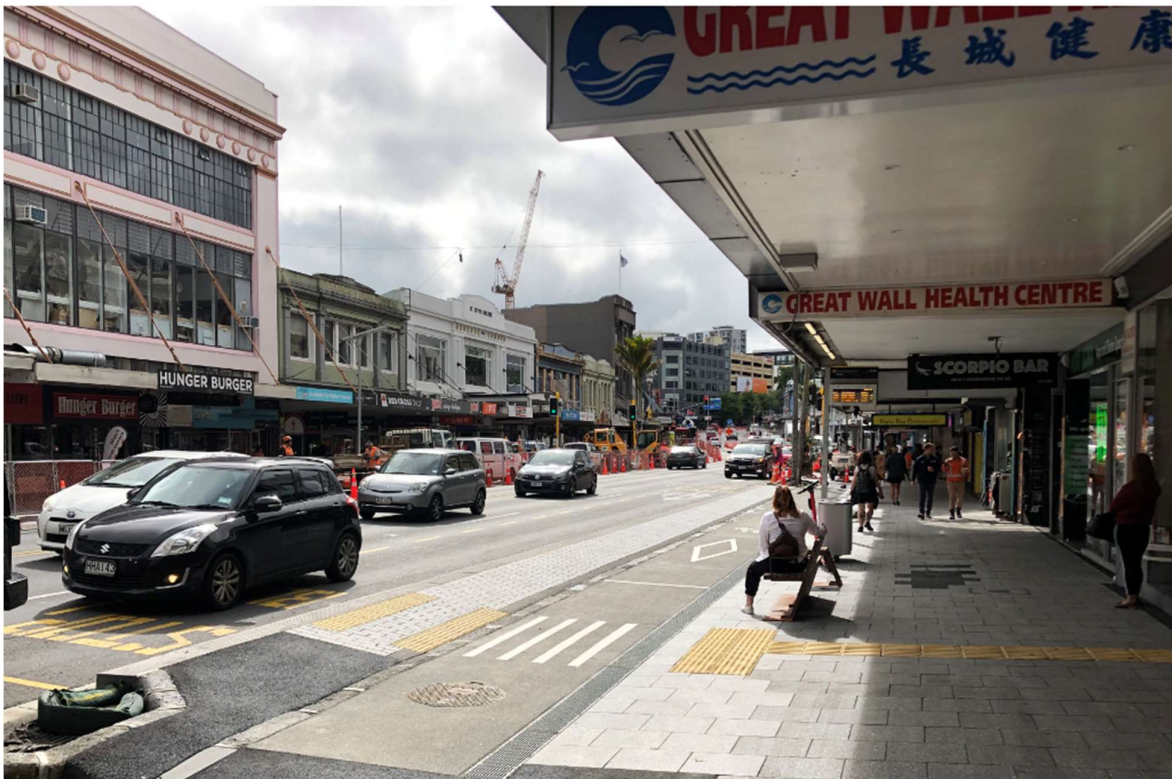
Figure 18: Example from Karangahape Road in Auckland (currently under construction)
