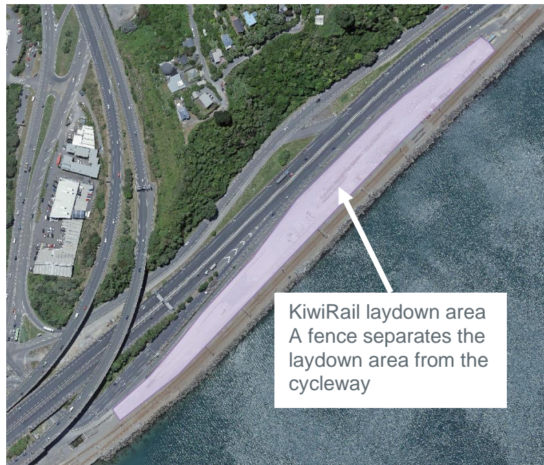
Figure 9: KiwiRail Laydown Area
