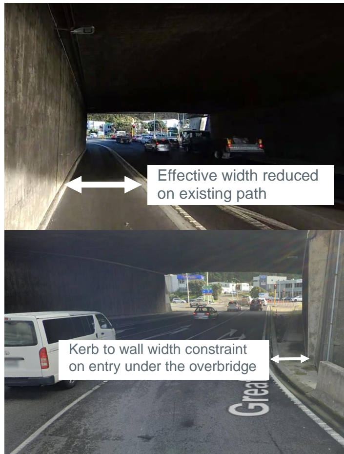
Figure 5: Width Constraints Under SH2 Overbridge
