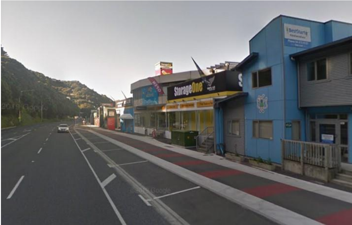
Figure 10: Indented P10 parking on Hutt Road (Source: Google Maps)
