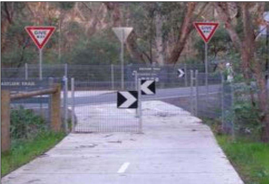
**Figure 13: Off-road path terminal treatments – staggered fence treatment**
