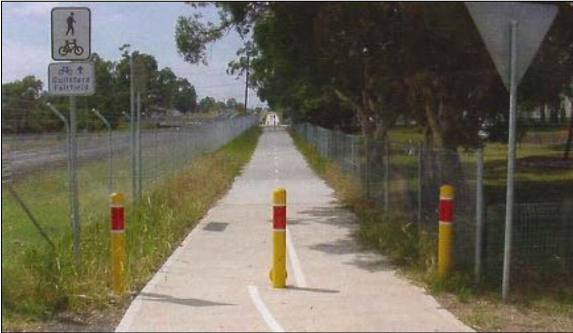
**Figure 12: Off-road path terminal treatments – bollard treatment**
