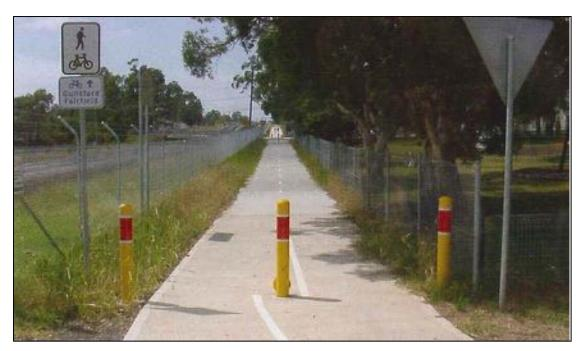
Figure 12: Off-road path terminal treatments - bollard treatment
