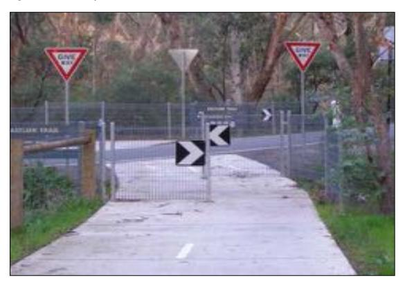
Figure 13: Off-road path terminal treatments – staggered fence treatment
