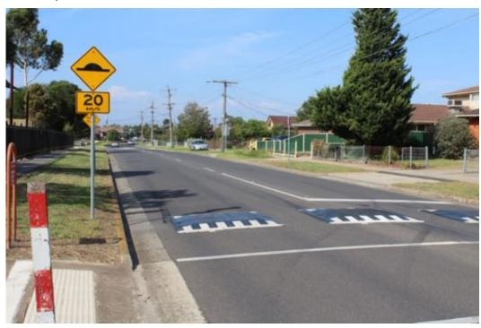
Figure 38: Example of a speed cushion
