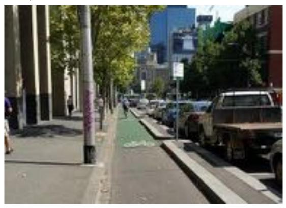
Figure 34: Example of green coloured pavement surfacing
